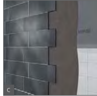
C Finally tile, or alternatively apply plaster.
