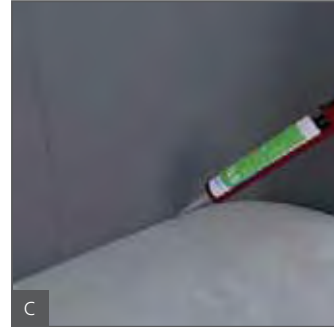
C Seal the open joints with wedi 610 adhesive and sealant, and reinforce the joints with wedi Tools reinforcement tape.
