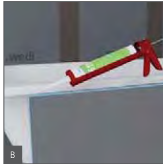
B ... glue and reinforce joints ...
