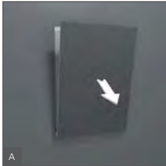
A Cut an appropriate recess in the wedi building board.
