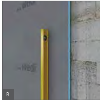
B Gently put up the building boards and align with a spirit level. Wait until the mortar has hardened and drill the holes in the wall.
