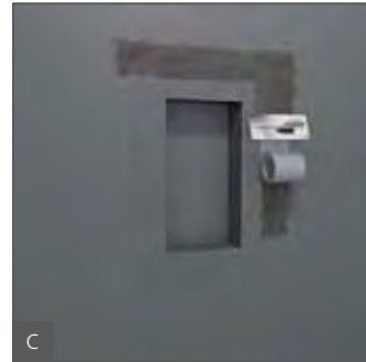
C Add sealant and wedi Tools sealant tape all round it.
