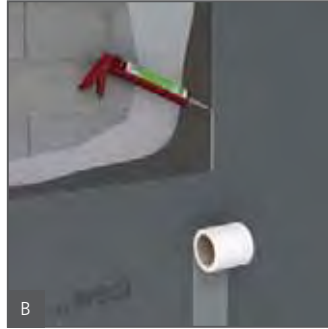
B Seal the joints with wedi 610 and apply wedi Tools joint reinforcement tape.
